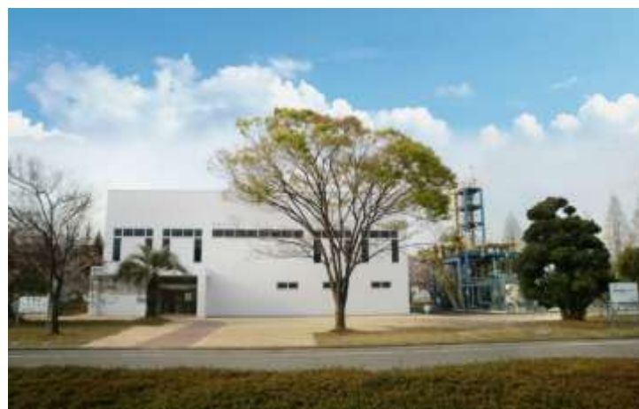
新TRC: New Operation Training Center
